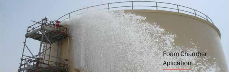
It is a fixed type foam fire-extinguishing system that is installed on the upper side of combustible oil storage tank and discharges the foam to the surface of fluid stored inside the tank in case of fire to separate oxygen from air. When the aqueous solution mixed with the foam agent is released through the orifice inside the foam chamber, the barrier film for preventing the backflow of oil mist ruptures and the low-expansion foam is generated by mixing the aqueous solution and the inhaled air.
