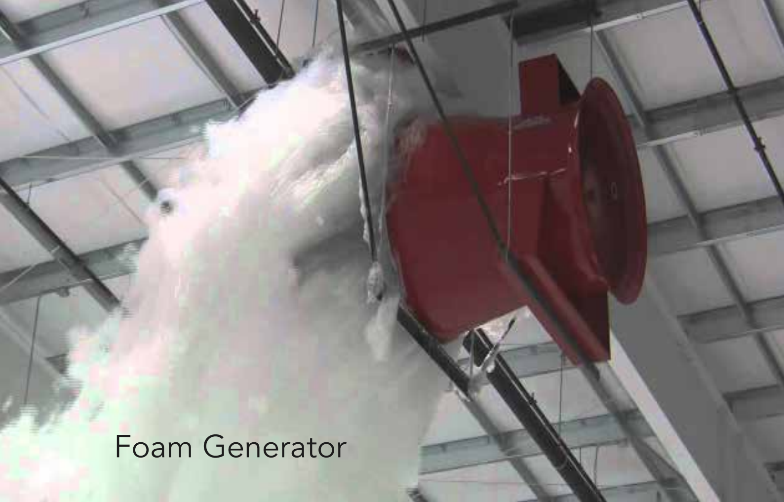
High Expansion Foam Generator
